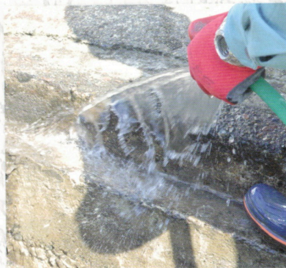
2 既存側溝の清掃
