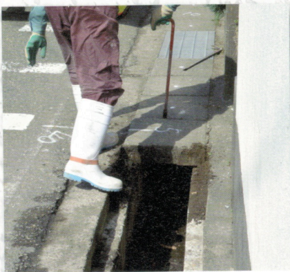
1 既存側溝の蓋撤去
